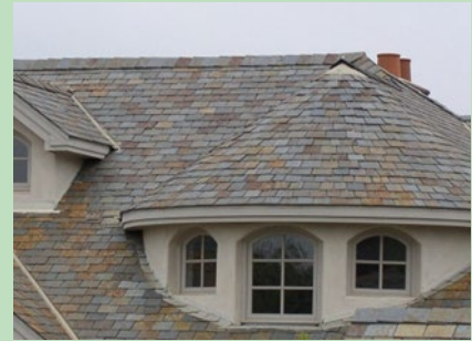
Slate tile Class "A" Roof
