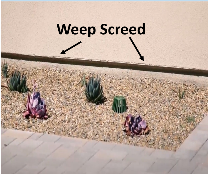
The weep screed serves as a vent so that moisture can escape the stucco wall finish just above the foundation.
